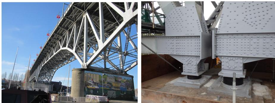
Figure 3. Granville Bridge: (a) elevation view, (b) replacement isolation bearings
